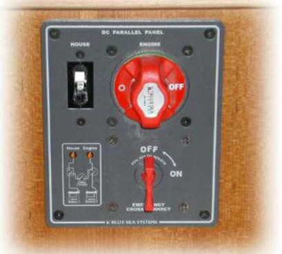
Battery cut-off switch for ultimate security and safety and emergency transfer switch if the need arises.
